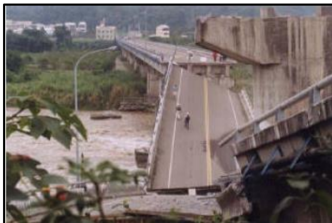
Figura 13. Colapso del Puente Shi-wei, Sismo Chi-Chi 1999 (National Institute of Standards and Technology, 1994)
