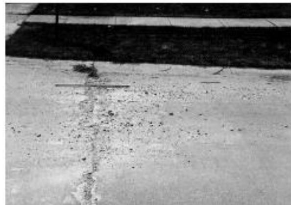
FIG. X2.1 Low Severity Blowup/Buckling
