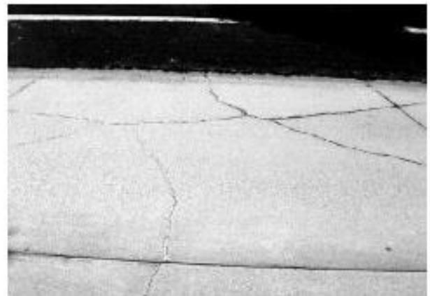
FIG. X2.8 Medium-Severity Divided Slab
