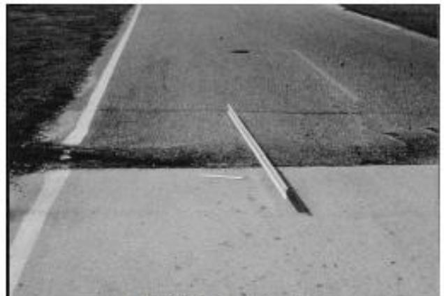
FIG. X1.46 High-Severity Shoving
