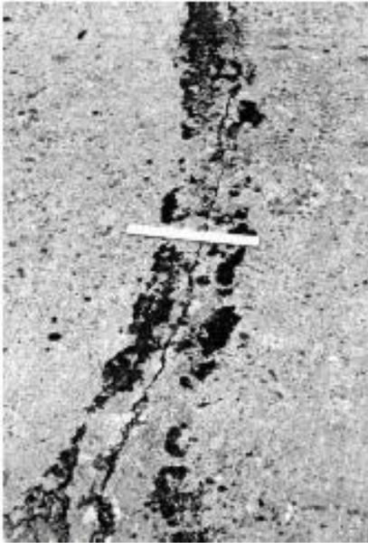
FIG. X2.22 Low-Severity Linear Cracking
