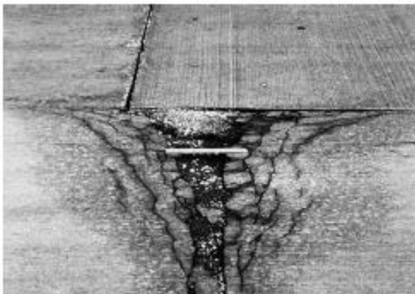
FIG. X2.11 Medium-Severity Durability Cracking
