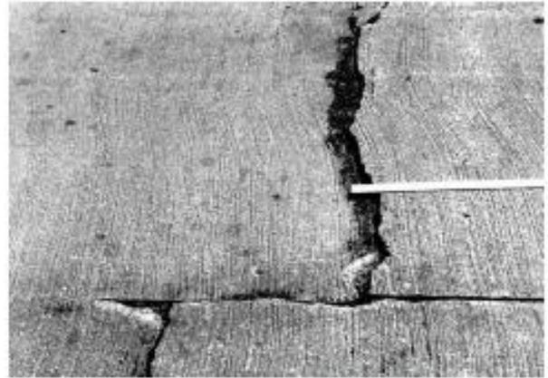
FIG. X2.24 High-Severity Linear Cracking
