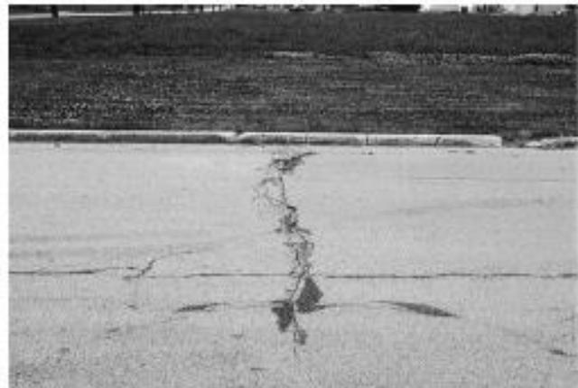
FIG. X1.30 High-Severity Longitudinal and Transverse Cracking
