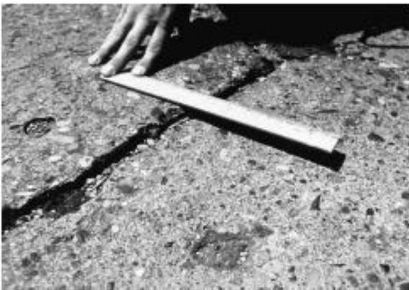
FIG. X2.14 Medium-Severity Faulting
