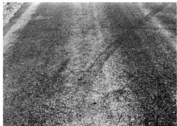
FIG. X1.4 Low-Severity Bleeding
