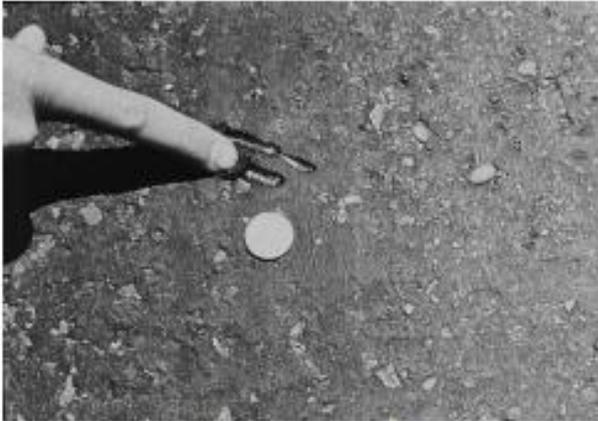
FIG. X1.5 Medium-Severity Bleeding
