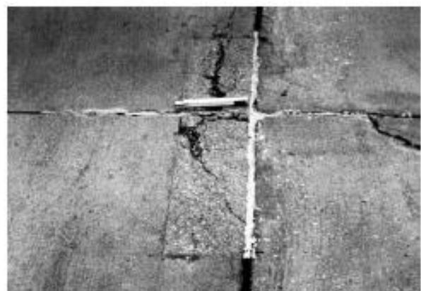
FIG. X2.30 High-Severity Patching, Small
