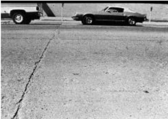
**FIG. X2.48 Low-Severity Spalling, Joint**
