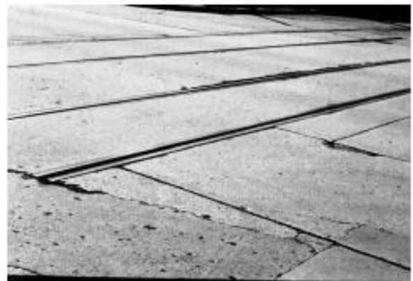
FIG. X2.38 Low-Severity Railroad Crossing
