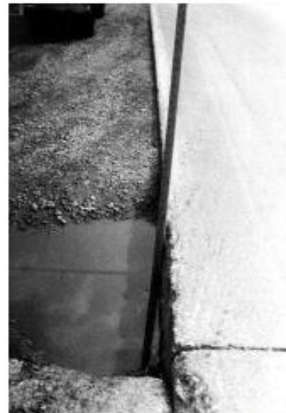
FIG. X2.21 High-Severity Lane/Shoulder Drop-Off
