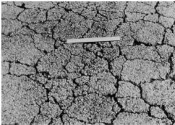
FIG. X1.3 High-Severity Alligator Cracking
