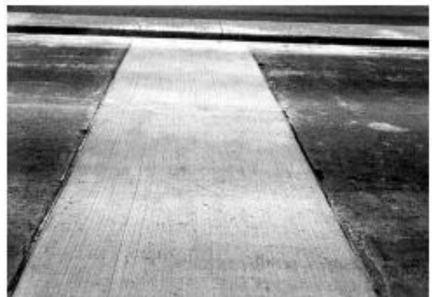
FIG. X2.25 Low-Severity Patching, Large and Utility Cuts
