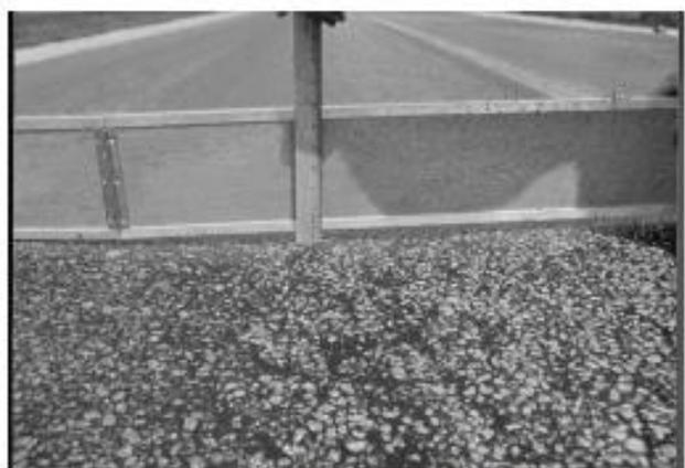
FIG. X1.42 Medium-Severity Rutting
