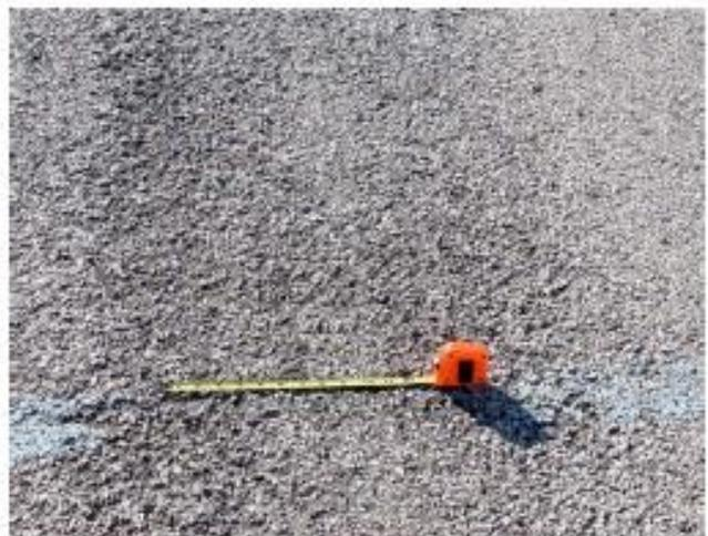
FIG. X1.51 Medium-Severity Raveling
