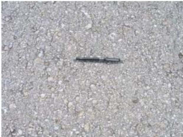
FIG. X1.53 Low-Severity Weathering (Surface Wear)
