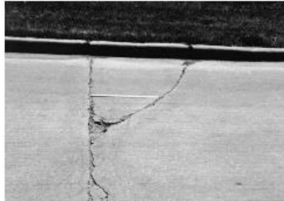
FIG. X2.5 Medium-Severity Corner Break
