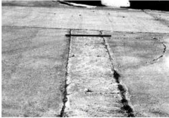
FIG. X2.26 Medium-Severity Patching, Large and Utility Cuts
