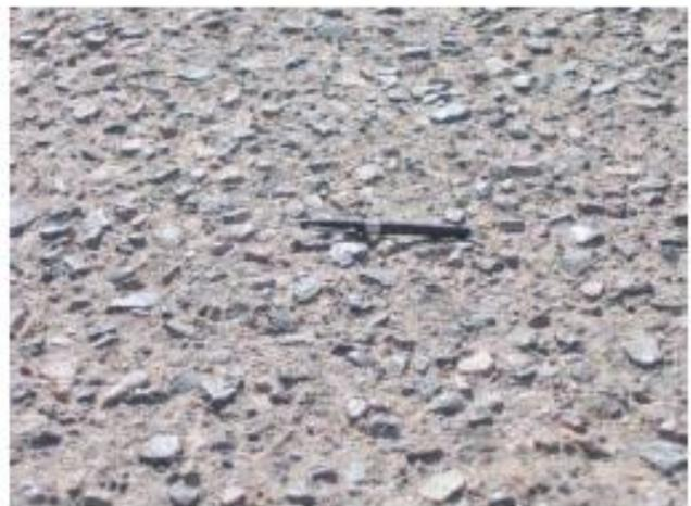
FIG. X1.55 High-Severity Weathering (Surface Wear)
