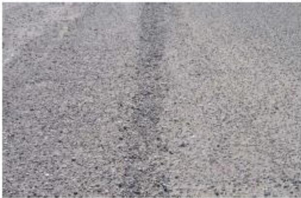
FIG. X1.52 High-Severity Raveling
