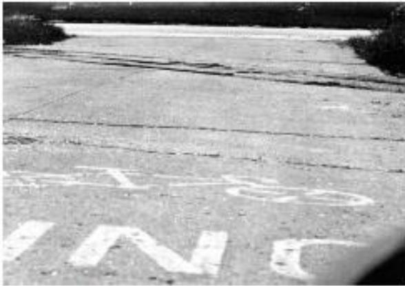
FIG. X2.39 Medium-Severity Railroad Crossing
