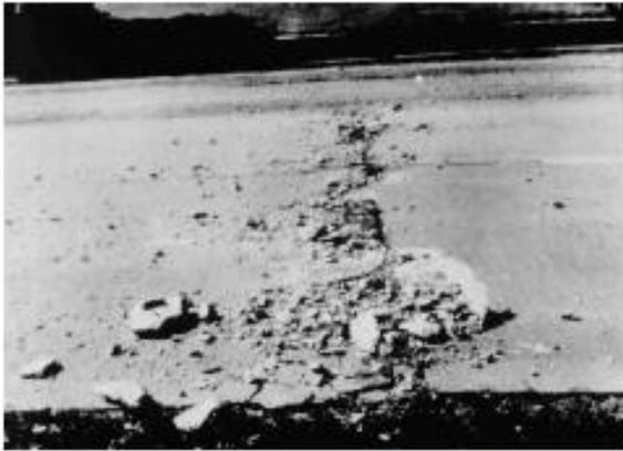
FIG. X2.2 Medium Severity Blowup/Buckling
