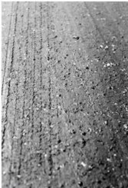
FIG. X1.6 High-Severity Bleeding
