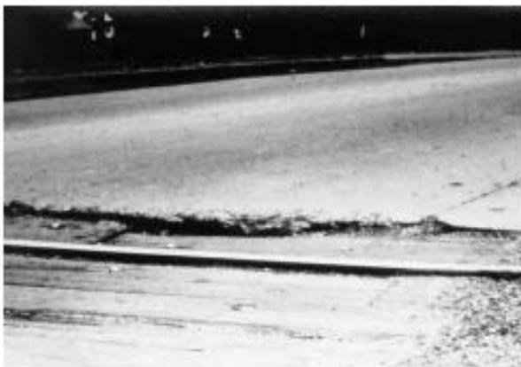
FIG. X2.40 High-Severity Railroad Crossing
