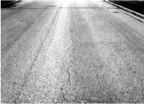
FIG. X1.1 Low-Severity Alligator Cracking
