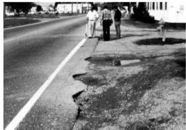
FIG. X1.21 High-Severity Edge Cracking
