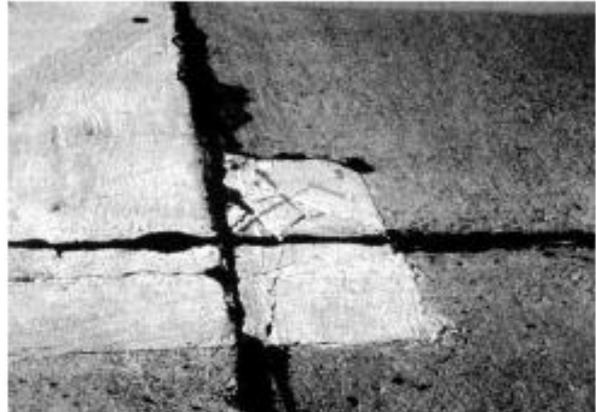
FIG. X2.29 Medium-Severity Patching, Small
