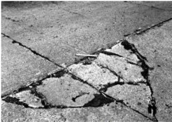
FIG. X2.6 High-Severity Corner Break
