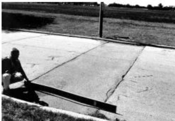
FIG. X1.32 Medium-Severity Patching and Utility Cut Patching
