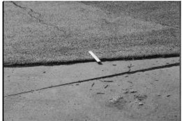
FIG. X1.45 Medium-Severity Shoving
