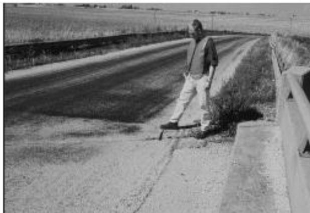
FIG. X1.44 Low-Severity Shoving
