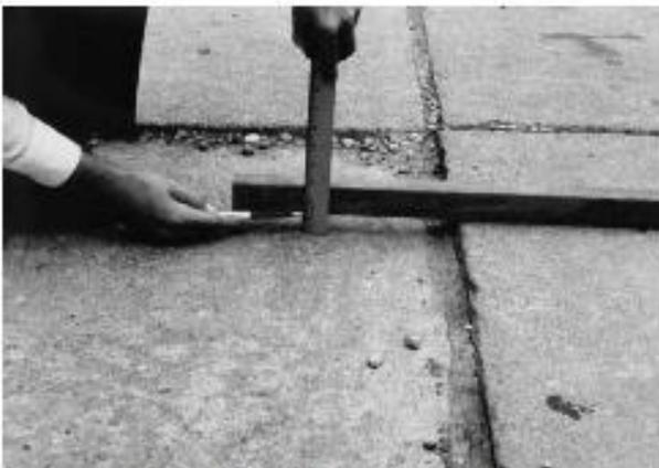
FIG. X2.15 High-Severity Faulting
