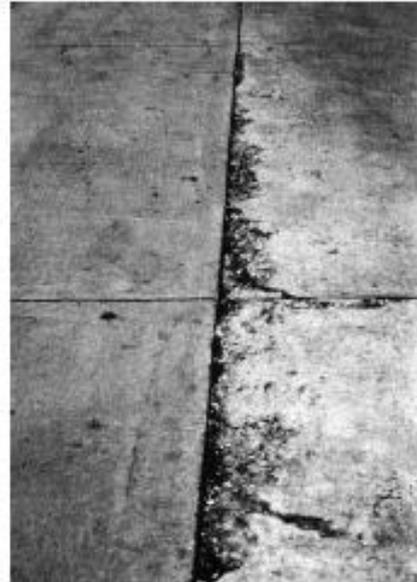
**FIG. X2.49 Medium-Severity Spalling, Joint**
