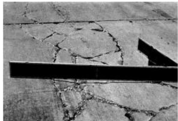
FIG. X2.37 High-Severity Punchout
