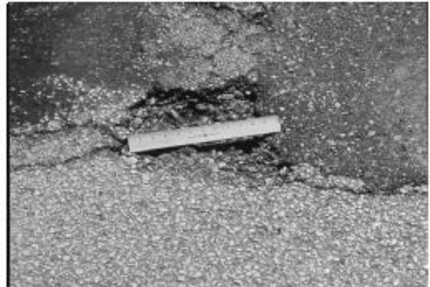
FIG. X1.35 Low-Severity Pothole
