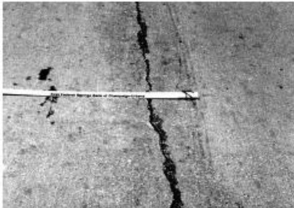
FIG. X2.23 Medium-Severity Linear Cracking
