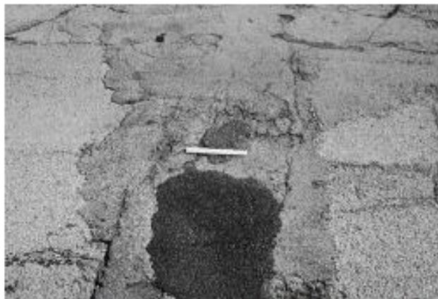
FIG. X1.33 High-Severity Patching and Utility Cut Patching
