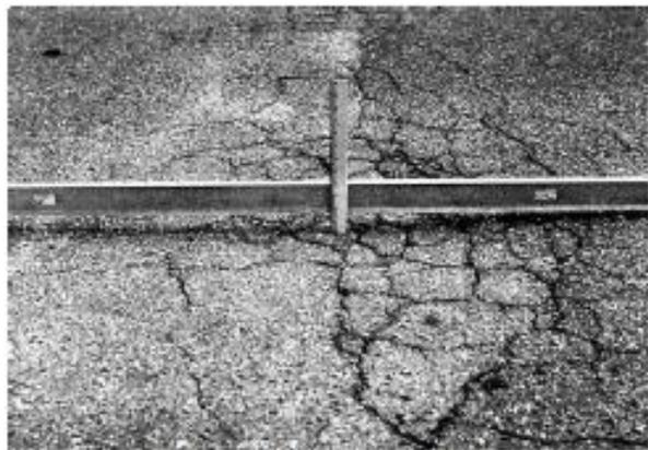
FIG. X1.18 High-Severity Depression
