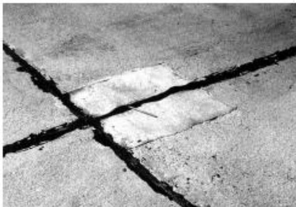
FIG. X2.28 Low-Severity Patching, Small
