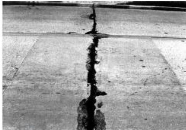
FIG. X2.16 Low-Severity Joint Seal Damage
