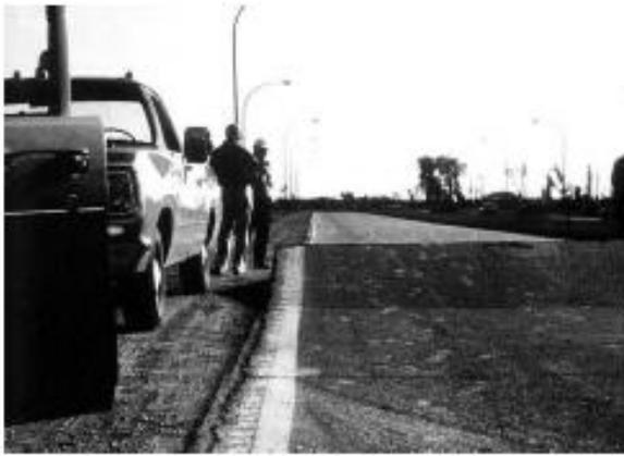
FIG. X2.3 High-Severity Blowup/Buckling
