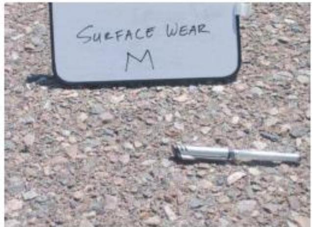
FIG. X1.54 Medium-Severity Weathering (Surface Wear)
