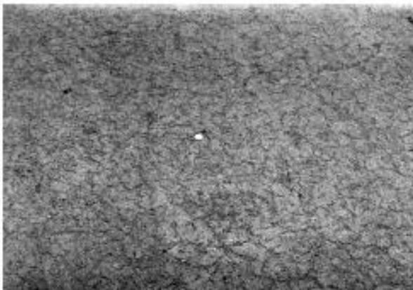
FIG. X2.41 Low-Severity Scaling, Map Cracking, and Cracking
