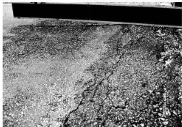
FIG. X1.12 High-Severity Bumps and Sags
