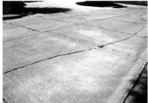
FIG. X2.7 Low-Severity Divided Slab
