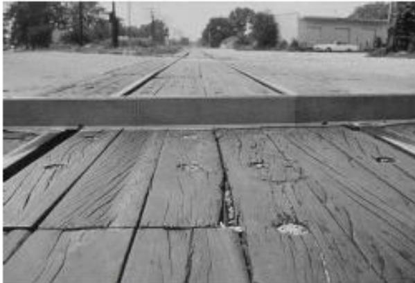
FIG. X1.38 Low-Severity Railroad Crossing
