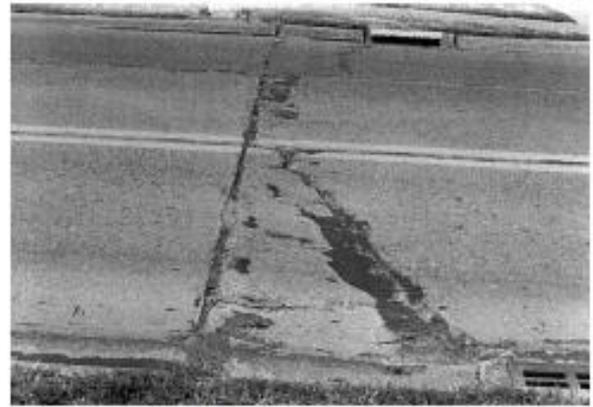
FIG. X2.36 Medium-Severity Punchout
