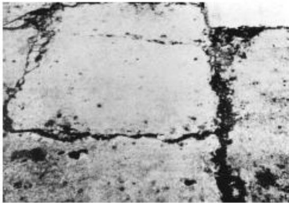
FIG. X2.27 High-Severity Patching, Large and Utility Cuts
