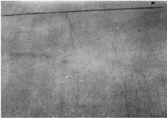
FIG. X2.44 Shrinkage Cracks
