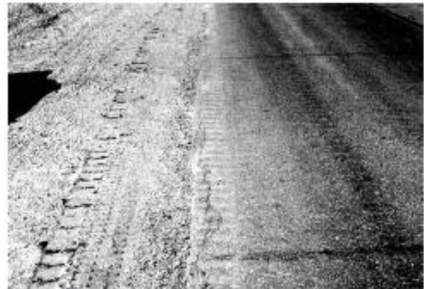
FIG. X1.22 Low-Severity Joint Reflection Cracking
