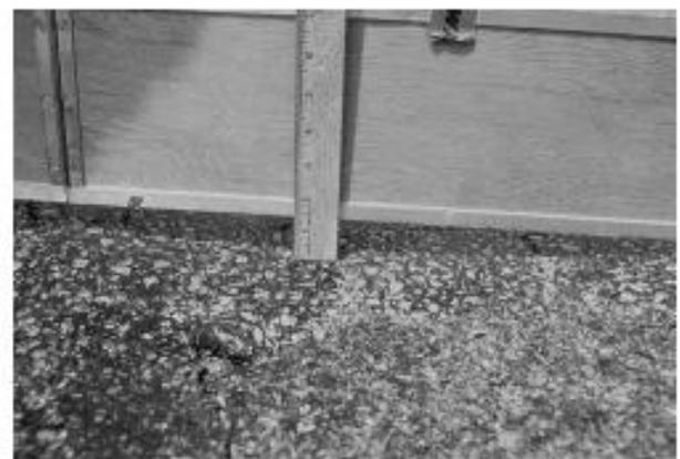
FIG. X1.43 High-Severity Rutting
