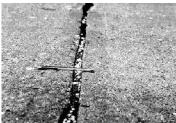
FIG. X2.18 High-Severity Joint Seal Damage
