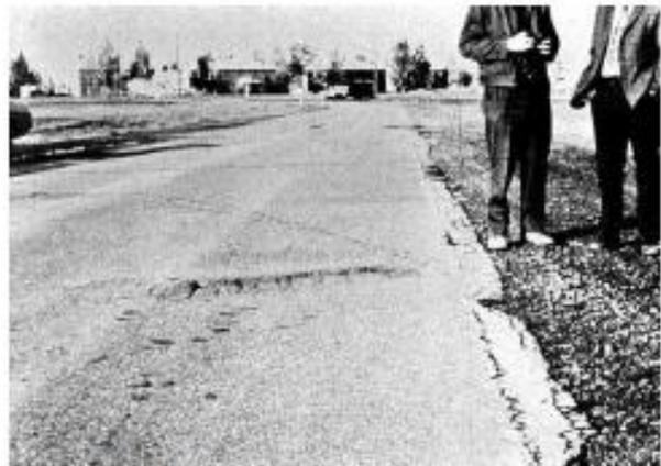
FIG. X1.11 Medium-Severity Bumps and Sags
