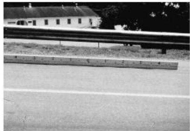
FIG. X1.13 Low-Severity Corrugation
