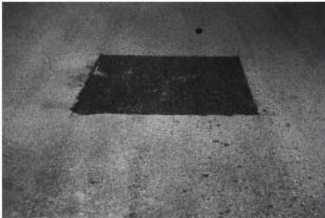
FIG. X1.31 Low-Severity Patching and Utility Cut Patching
