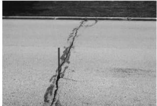
FIG. X1.29 Medium-Severity Longitudinal and Transverse Cracking
