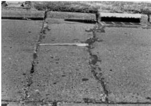
FIG. X2.35 Low-Severity Punchout
