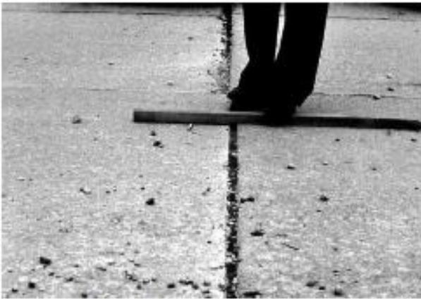
FIG. X2.13 Low-Severity Faulting
