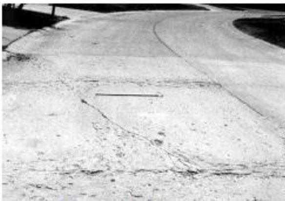
FIG. X2.12 High-Severity Durability Cracking
