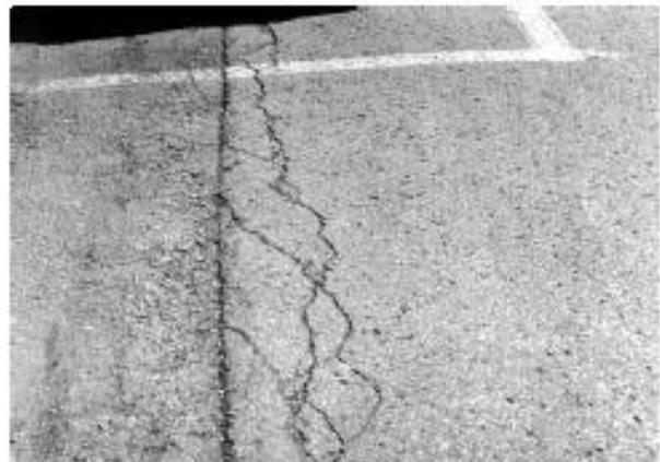
FIG. X1.20 Medium-Severity Edge Cracking
