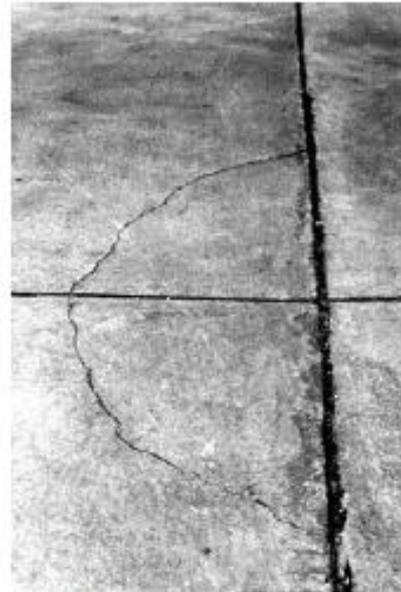
FIG. X2.4 Low-Severity Corner Break
