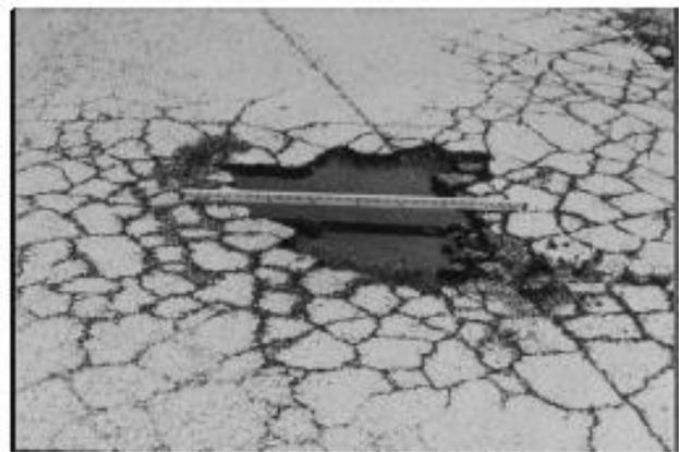
FIG. X1.37 High-Severity Pothole
