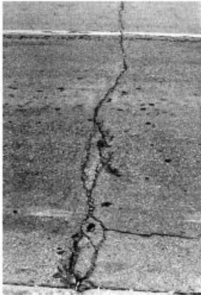
FIG. X1.23 Medium-Severity Joint Reflection Cracking
