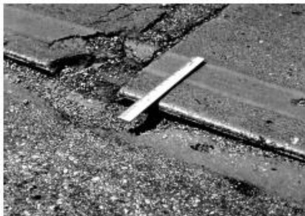
FIG. X2.19 Low-Severity Lane/Shoulder Drop-Off
