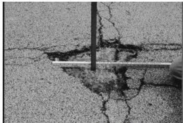
FIG. X1.36 Medium-Severity Pothole
