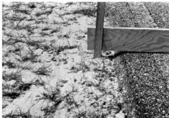
FIG. X1.25 Low-Severity Lane/Shoulder Drop-Off
