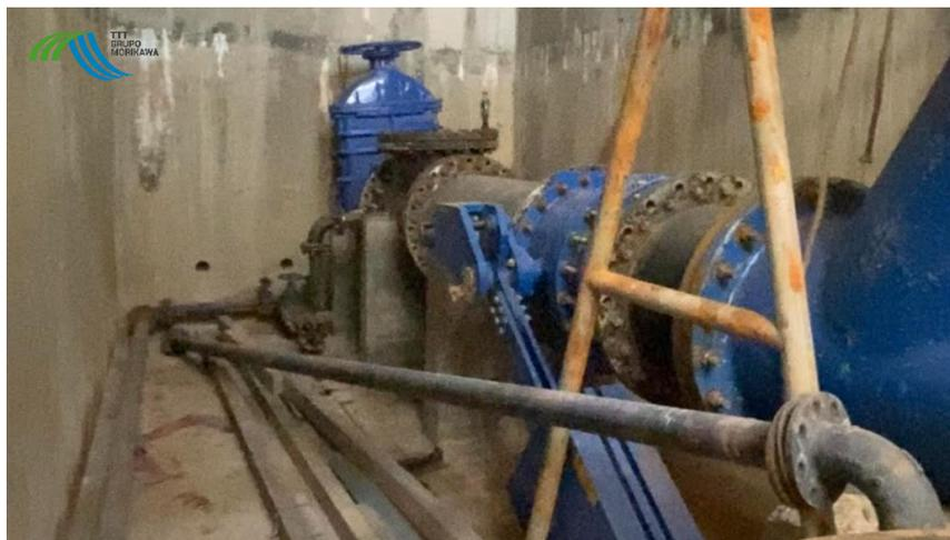
IMAGEN 2: INTERIOR CÁMARA DE VÁLVULAS SUBTERRANEA, LAGUNA ACUCOCHA / FUENTE: PROPIA
